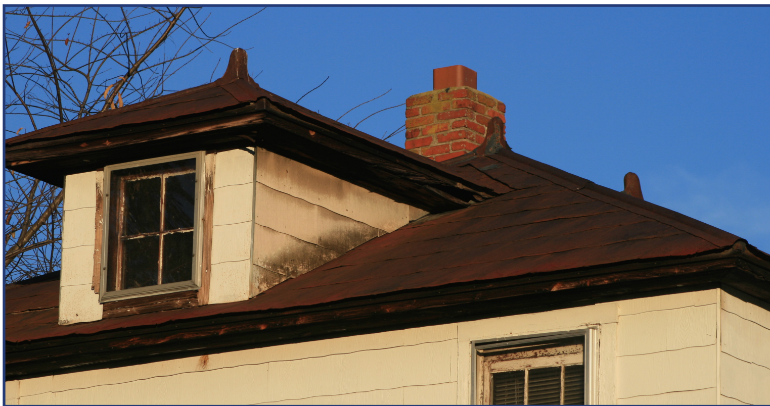
Figure 8. Dent-Brooks House Roofline
